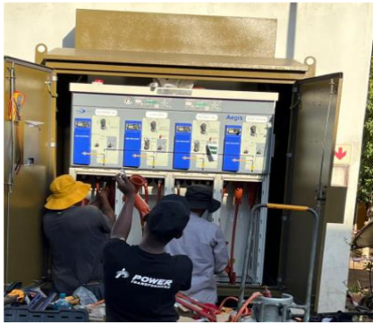
Swellendam, Replacement of Old redundant MV oil switchgear, R 507 993,00
