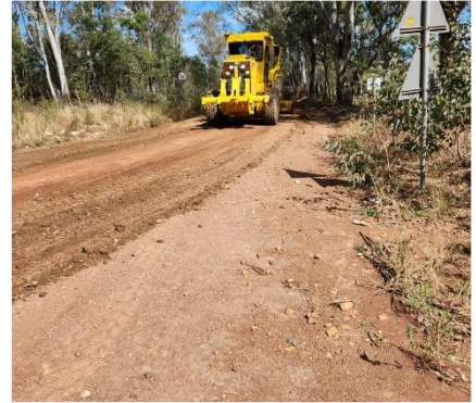
Swellendam: Gravel Road Upgrade: R 1 524 350,00
