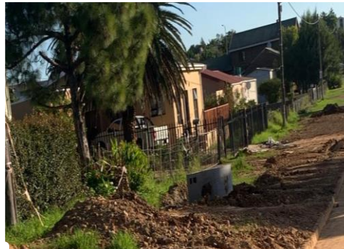
Railton sanitation upgrade, street front sewers: R 1 300 000,00
